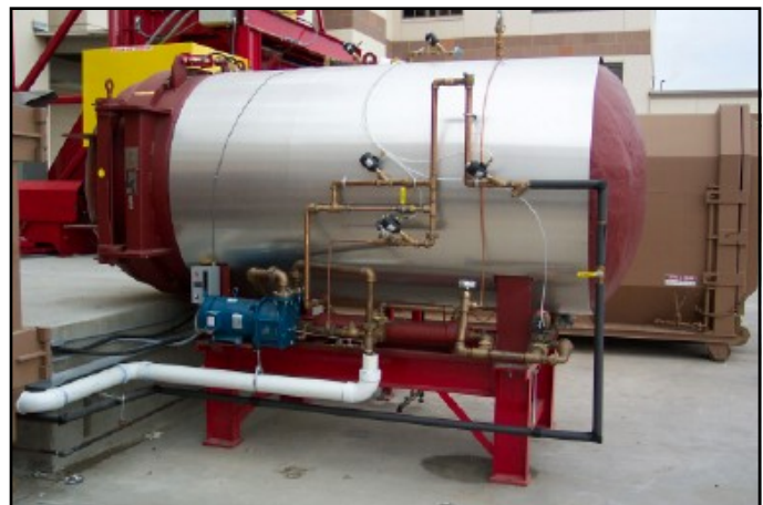
Autoclave technology uses heat, steam and pressure to sterilize every load in about 20 minutes.
